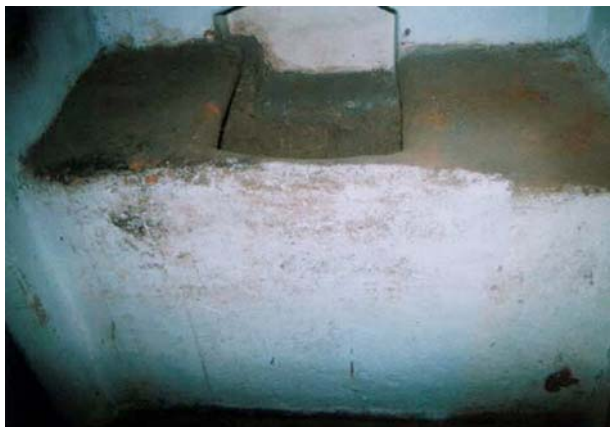
Figure 2. Mankattai (Mud house), 1.5 m height, 1.5 m width, 2 m length, capacity > 500 Kg.
